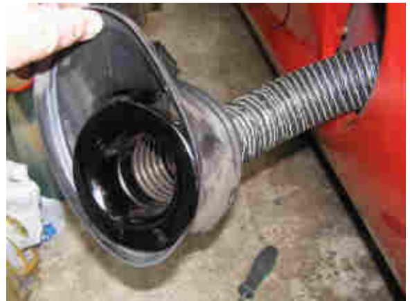
Flexi duct fitted through inner liner
